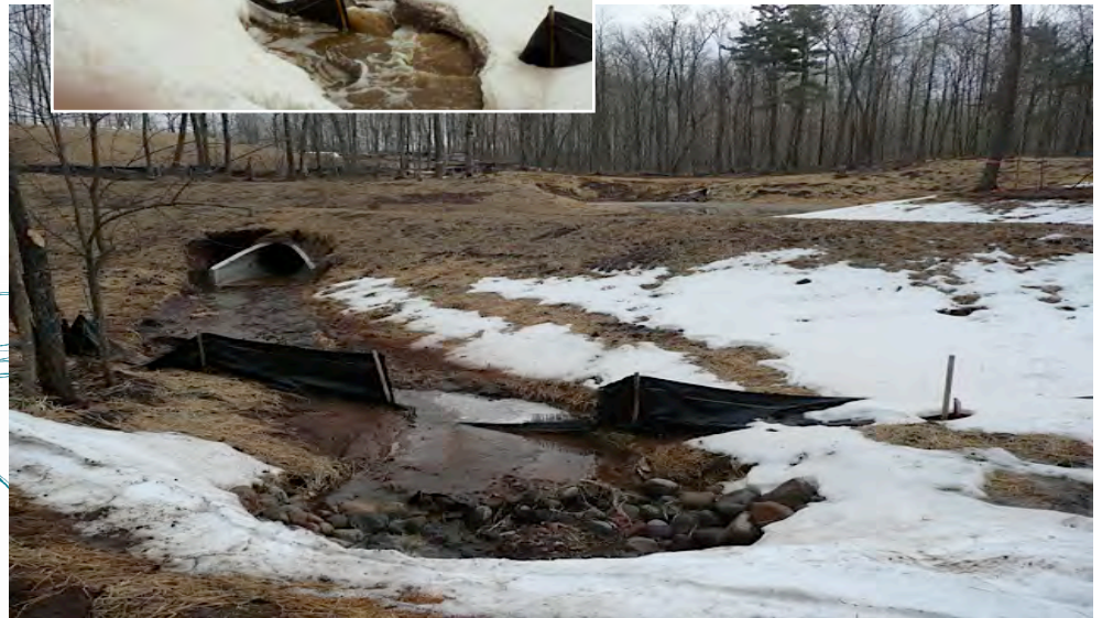
Below: Outlet pipe on March 29.
