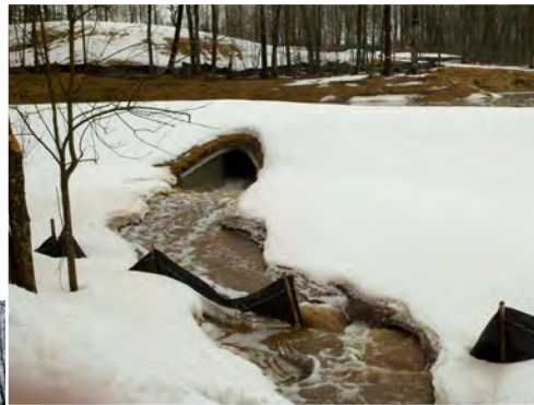
Left: March 12: Outlet pipe with water flowing out of the basin
